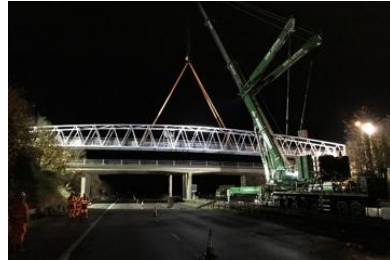
Warren truss bridge at Tithebarn, Exeter being craned into place over the M5
