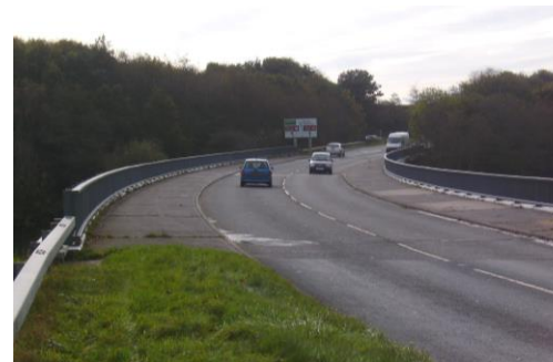
Existing Deep Lane Bridge
